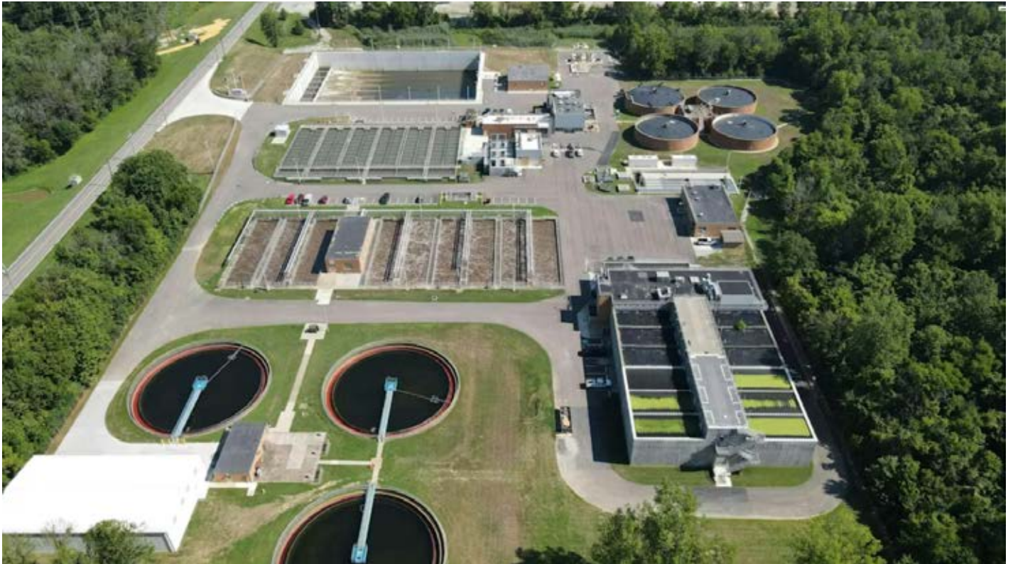
An aerial view of the Evansville West Wastewater Treatment Plant.
