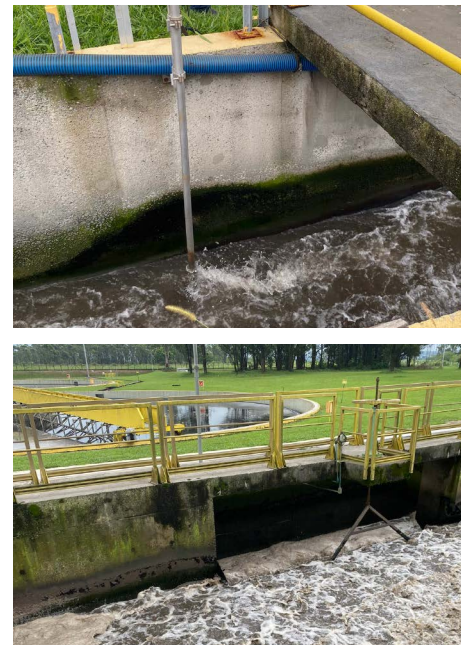
Figure 2 - SENTRY Wastewater quality monitoring sensors uniquely placed in the WWTP's sewage channel influent
