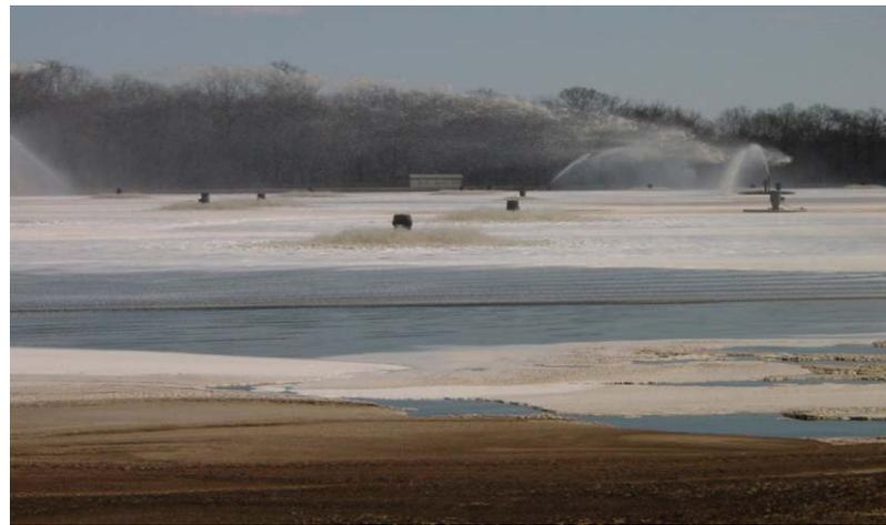
Figure 1: Aerated Stabilization Basin (ASB) Treatment System
