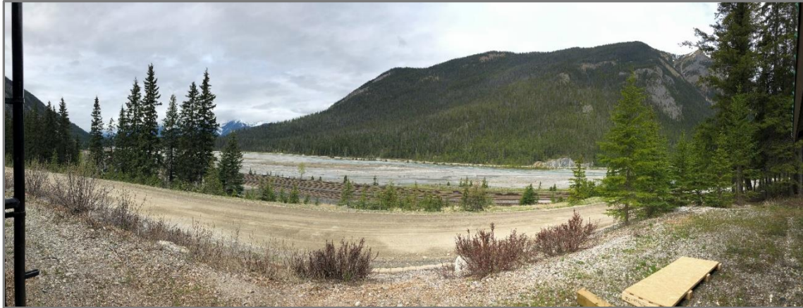
Figure 1 Remote MBR wastewater treatment plant location in Yoho Park, British Columbia, BC.
