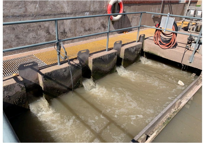
Figure1: Sensors installed at primary influent
